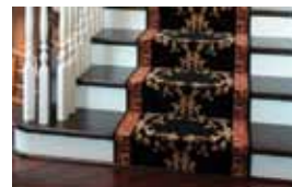
Open tread stairway, wood exposed both ends, carpet
